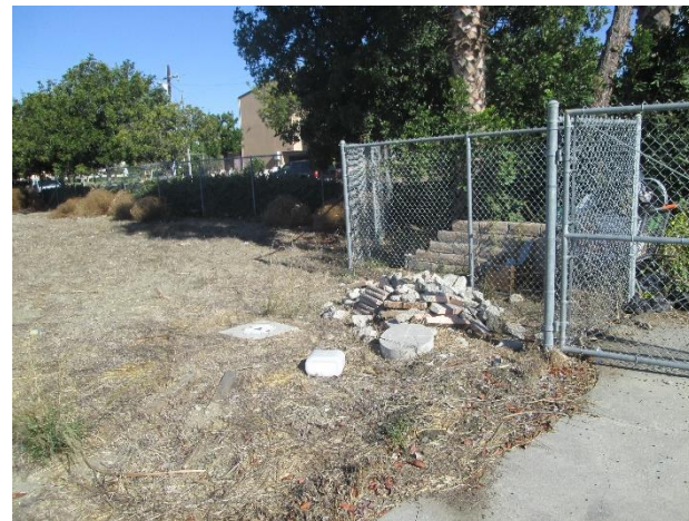
9. Typical debris and groundwater monitoring well.
