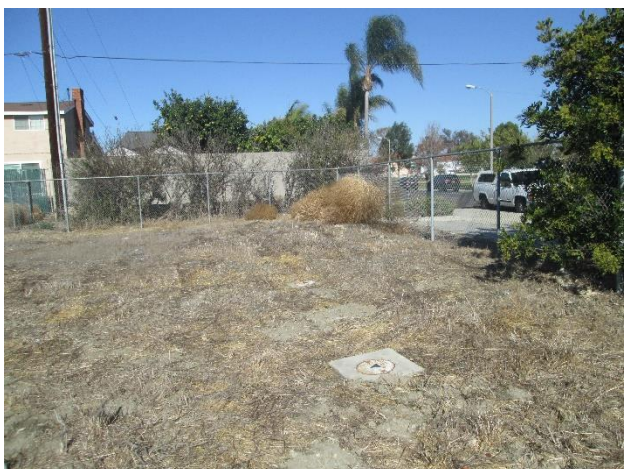
10. Typical groundwater monitoring wells.
