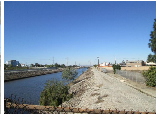
24. Western adjacent channel.
